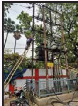
DTR Maintenance work.
