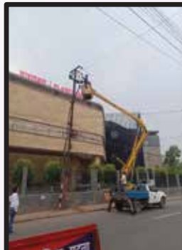
Road crossing dismanteling at Taramandal.
