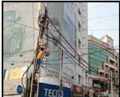
Removing downside network near Harinivas
